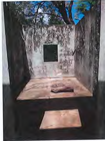
Figure 2.23 Internal detail of room. (Source: Acker Pty Ltd, 2017)
