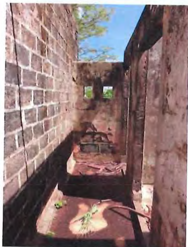
Figure 2.20 Internal detail of corridor. (Source: Acker Pty Ltd, 2017)
