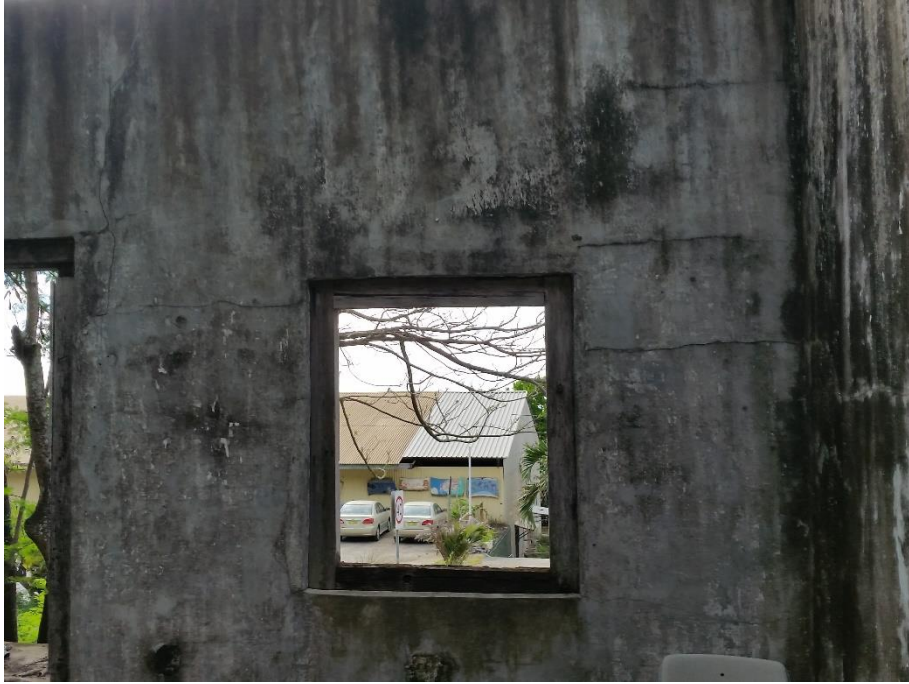
7. Front wall (internal view)
