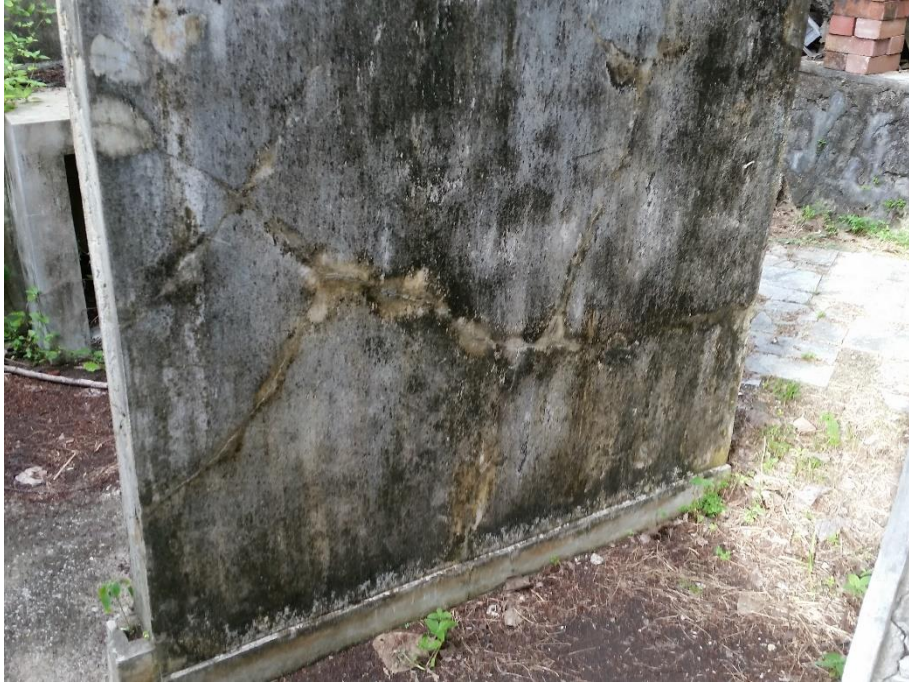
9. Wall cracking
