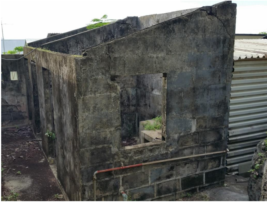
5. Rear wall of smaller unit
