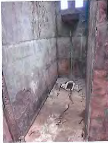
Figure 2.22 Internal detail of toilet. (Source: Acker Pty Ltd, 2017)
