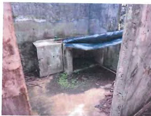
Figure 2.19 Internal detail of room. (Source: Acker Pty Ltd, 2017)
