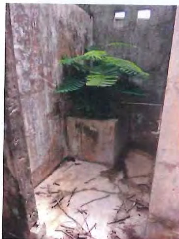
Figure 2.21 Internal detail. (Source: Acker Pty Ltd, 2017)
