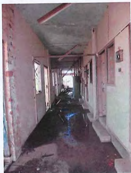
Figure 2.10 Looking north along the ground floor corridor. (Source: Acker Pty Ltd, 2017)
