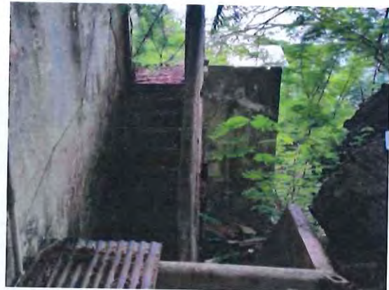
Figure 2.7 Northern stairs, first floor. (Source: Inter Engineering, 2018)
