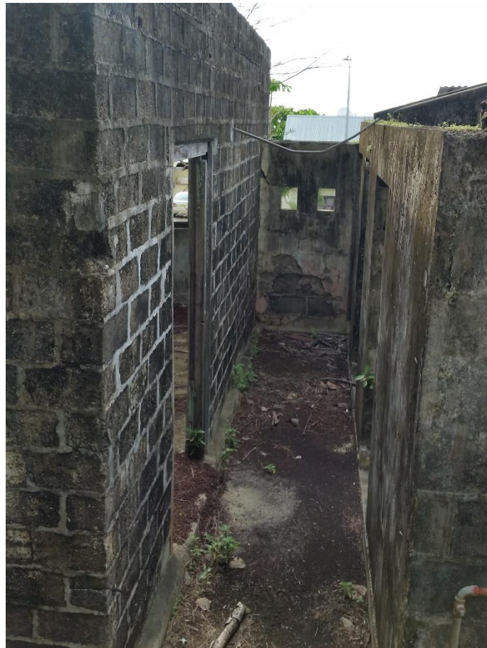
4. Corridor from rear
